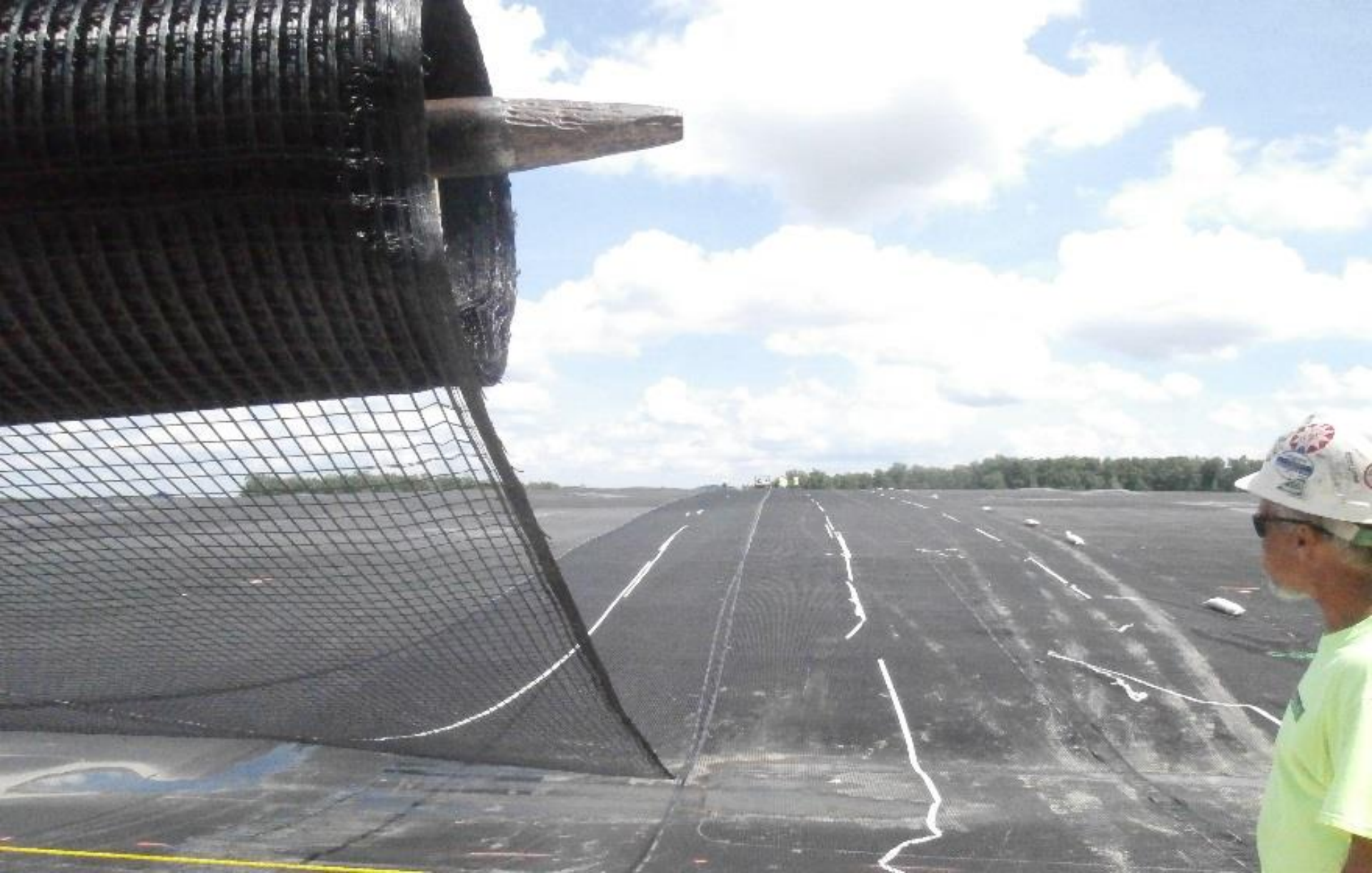
Deploying secondary geogrid over IRP cover
