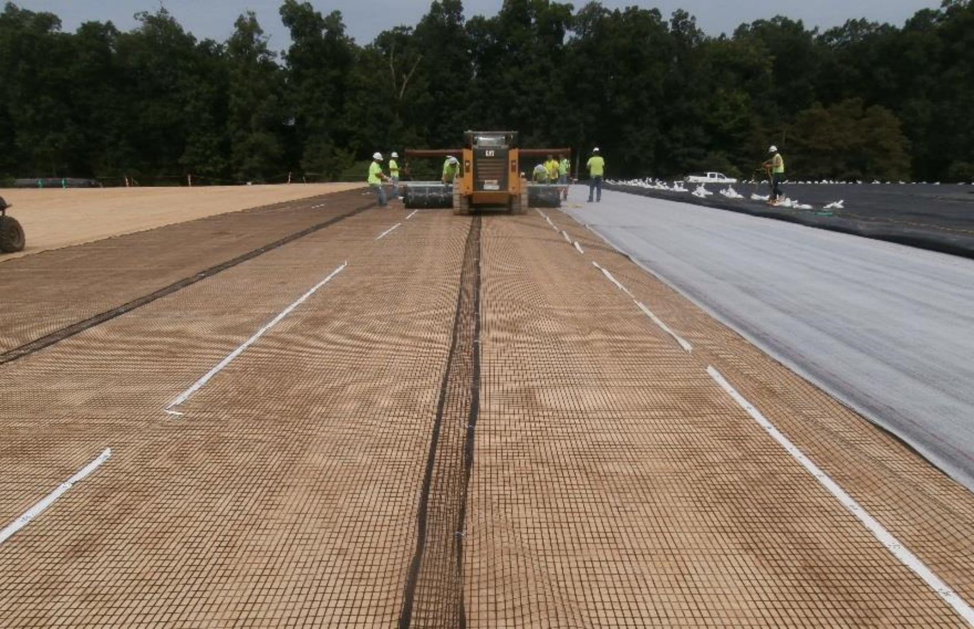
Deploying primary geogrid over leveling fill
